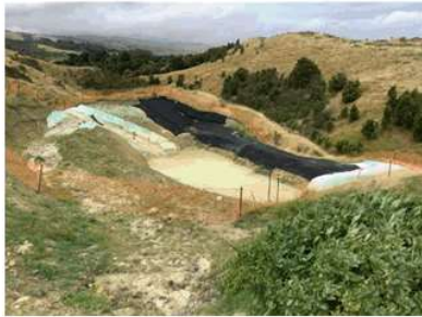
DECANTING EARTH BUND DEB 4 CATCHMENT
