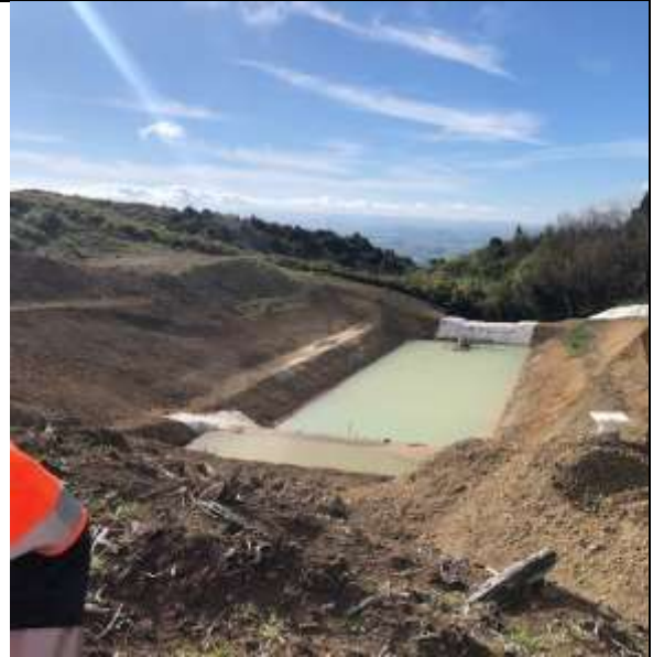
Figure 8. Chemically dosed sediment retention pond
