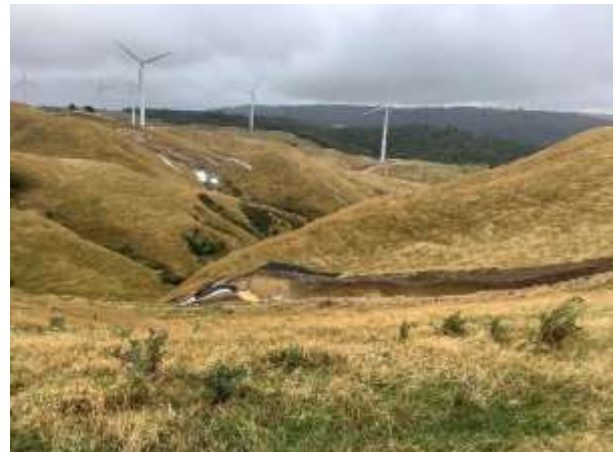
Figure 3. Sediment retention ponds in Construction Zone 2
