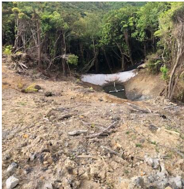
Figure 9. Decanting Earthbund installed in steep terrain
