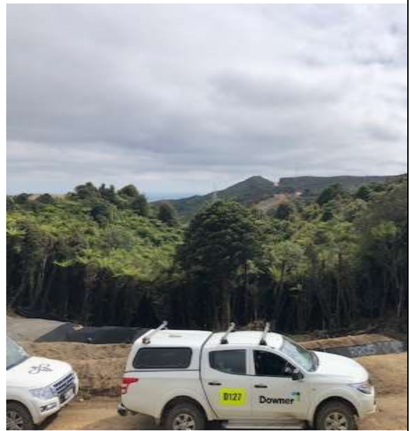
Figure 10. looking along southern access track/road
