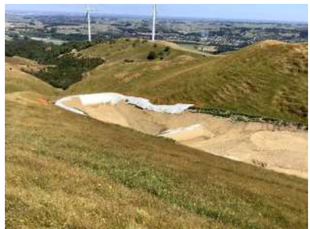
Figure 5. Sediment retention Pond in Construction Zone 2.
