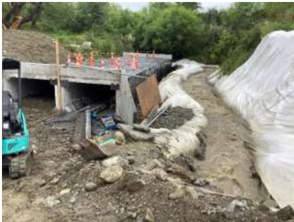
Figure 2. Temporary diversion as culverts are constructed off-line
