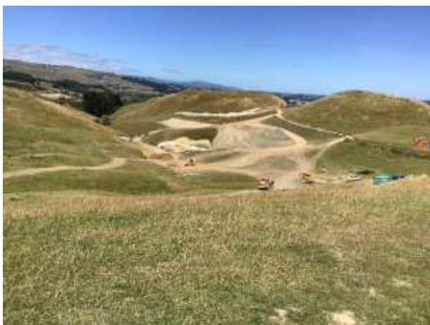
Figure 4. overview of construction Zone 1
